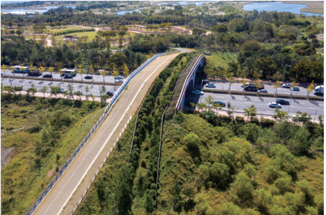
Figure 19. Ecological Bridge on Eulsukdo
